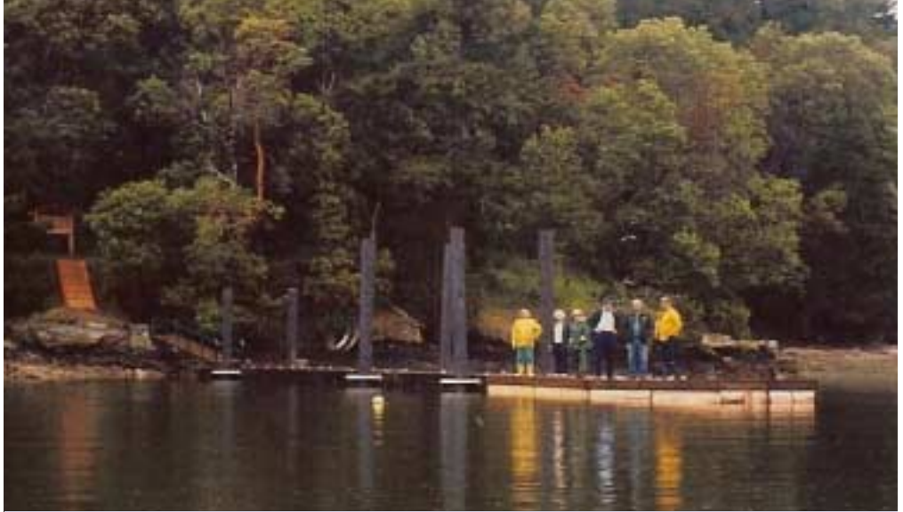
The dock in 1985 after the Army Engineers drove pilings etc
